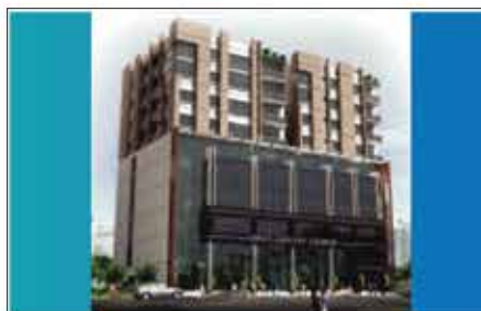
Haji Salim Tower Location : Chalkbazar Brand : Gree
