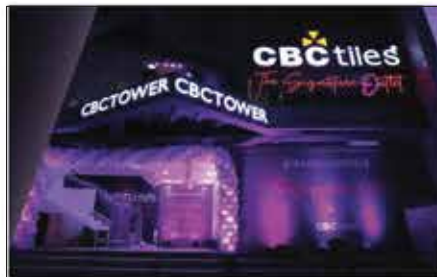
CBC Tower Location : Hatirpool Brand : Daikin
