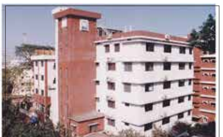
Monowara Hospital Location : Siddeshwari Road Brand : Midea
