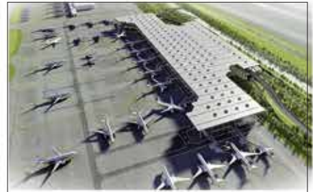
Airport 3rd Terminal(Extension) Location : Airport Brand : Samsung
